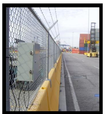
Southwest Microwave's MicroPoint™ Cable system pinpoints fence cut or climb attempts to within 3m, while ignoring environmental disturbances like wind, rain or vehicle traffic.
